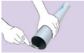
3. Deburring and chamfering
